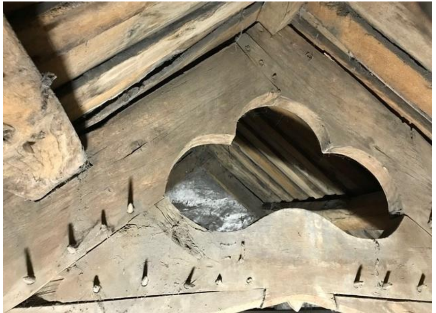
Caenog Roof over principal chamber with rebated boards between the rafters, a very rare feature Tree-ring dated to 1550
