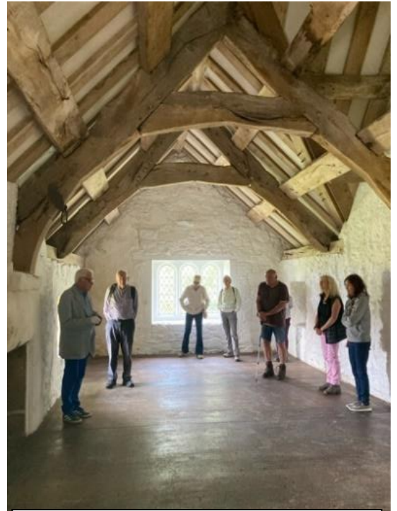
Upper Floor, Hafoty
