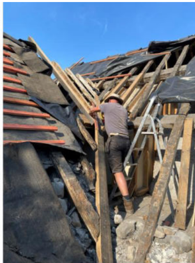
Repairs in reclaimed oak to the roof valley timbers
