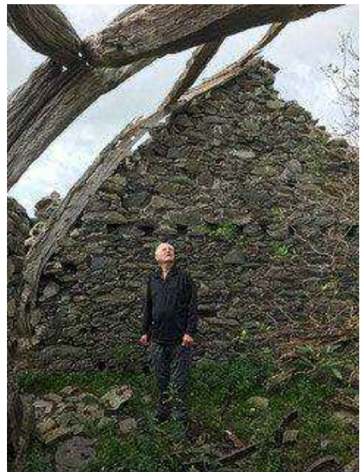
Hafotty Llanegryn. Two pairs of full cruck trusses survive (one blade has fallen and the roof is not too stable!); this room was originally open but floored over when the wall behind our treasurer was built (see the socket holes for the joists).
