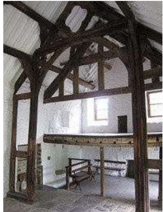
Penarth-fawr, near Criccieth. Built at some time after 1476. The so-called 'spere truss' echoes the aisled halls of the princes.
