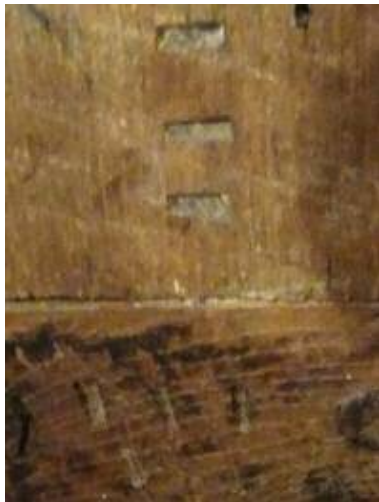
Carpenter's assembly marks Marciau adeiladu saer
